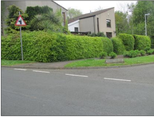
Entrance to Tern Court, missing drop kerbs on both sides of Collydean Way, with parking bays and bins creating an additional obstacle for pedestrians crossing to the west side of the road.
