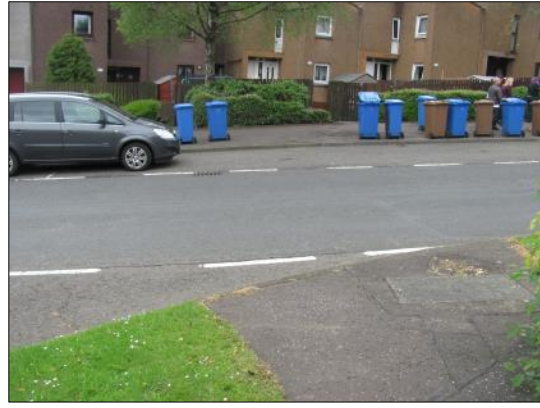
Entrance to Tern Court, missing drop kerbs on both sides of Collydean Way, with parking bays and bins creating an additional obstacle for pedestrians crossing to the west side of the road.
